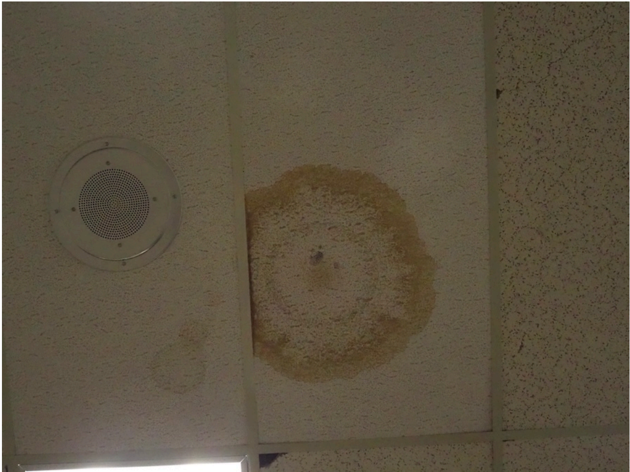
Water damage is visible in the ceiling tiles throughout the Beekman Center in Lansing on Jan. 29, 2026. (Anna Liz Nichols for ELi)
